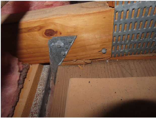
Roof to wall attachment - Clips
