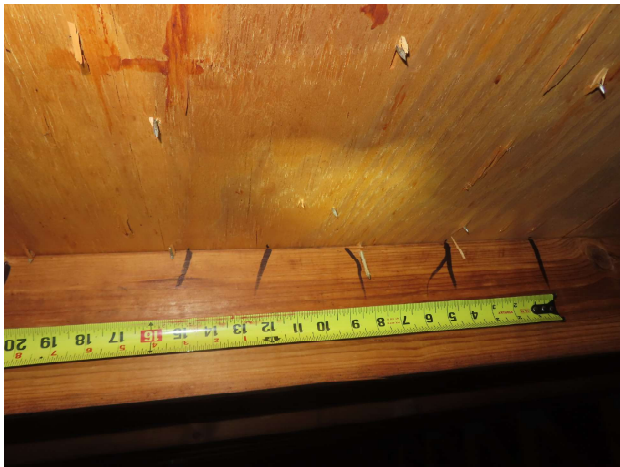
Roof deck nail spacing - Field
