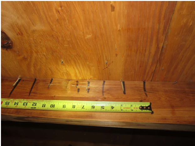
Roof deck nail spacing - Edge
